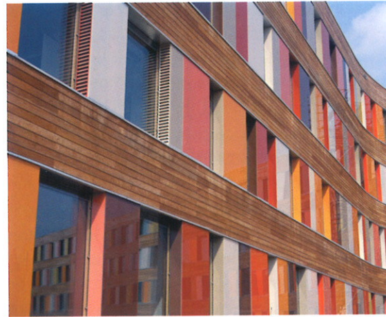
10 | View of the external building envelope with air intake vents, Federal Environment Agency, Sauerbruch Hutton, Dessau, Germany, 2005
