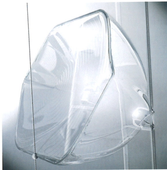
5 | The facade's modules are made of borosilicate glass and attach to a glass tubular structural system.
