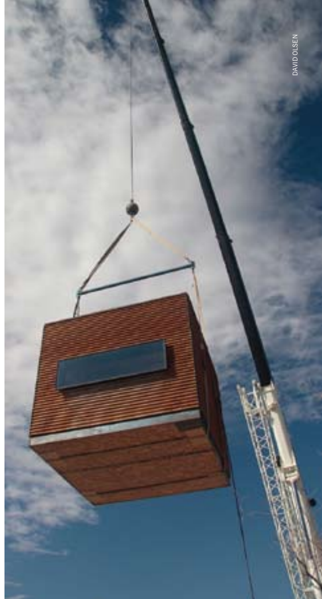
A SEED[pod] house is hoisted into place.
