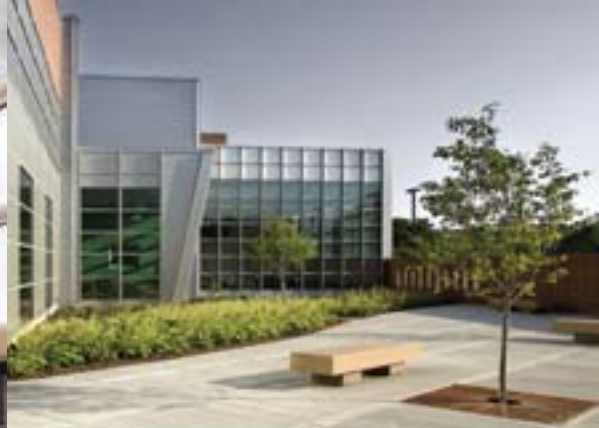
RicciGreene Associates, headed by Pratt alumnus Ken Ricci, used a “thin” design that is only one room deep with a security enclosure composed of the building perimeter, thereby eliminating the need for high security fencing.
